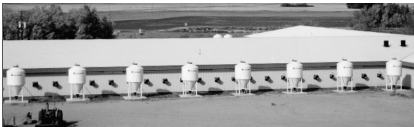
Ventilation at the PSC Elstow research barn features both sidewall and chimney outlets.
