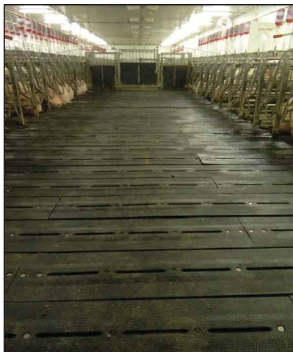
Figure 1. Rubber slats installed in an I-pen.
