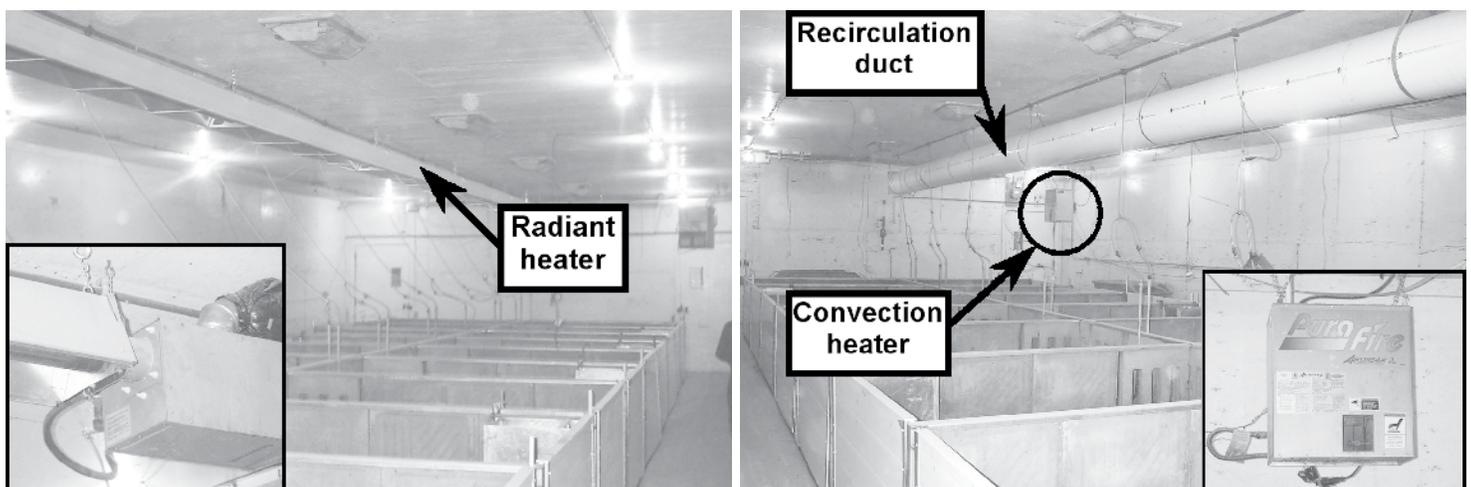
**Figure 1.** Photo of the experimental rooms. A: Treatment room with a 50-ft long infrared radiant heater (inset- heater part); B: Conventional production room with a forced-air convection heater (inset).
