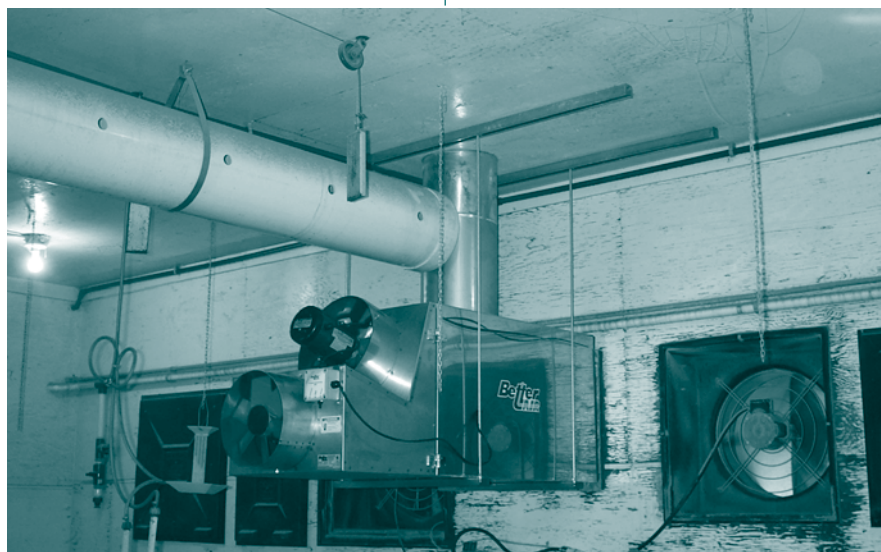
Figure 1. Heat exchanger installed in a grow-finish room.
