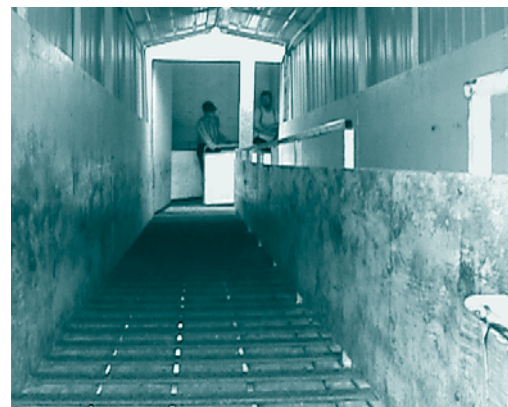
Figure 1. Hydraulic loading ramp with manway (looking down ramp from truck entry).
