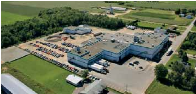
An aerial view of the Olymel Yamachiche plant. Photo courtesy Olymel.
