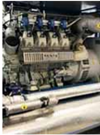
The CHP unit efficiency uses clean-burning natural gas to run an engine that creates power and recovers waste heat. The system is kept stable by using a combination of temperature-regulating inputs and outputs.
