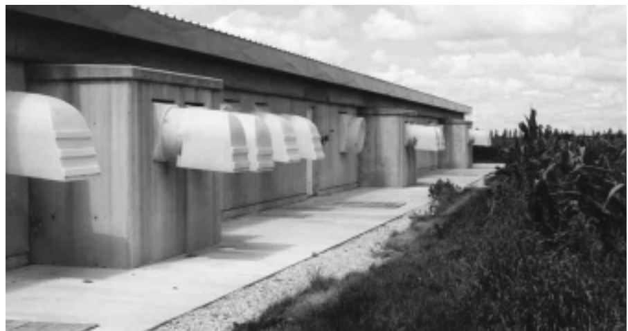
Figure 1: Fan arrangement and manure pit design along the sidewall of the concrete barn built by FRED GROENESTEGE CONSTRUCTION LIMITED (Sebringville, ON).
