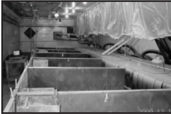
The EDA design implemented at PSCI and tested with full strip curtains
