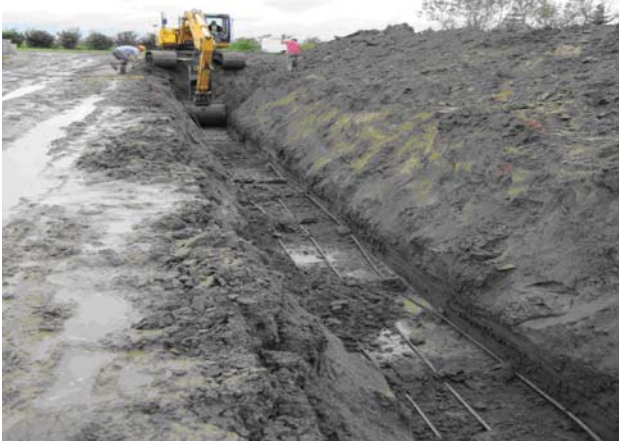
Figure 2. (LEFT) Installation of pipes for the ground source heating system installed in a grow-finish room. (RIGHT) in-room heat pump connected to ground source heat system
