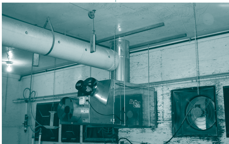
Figure 1. Heat exchanger installed in a grow-finish room.
