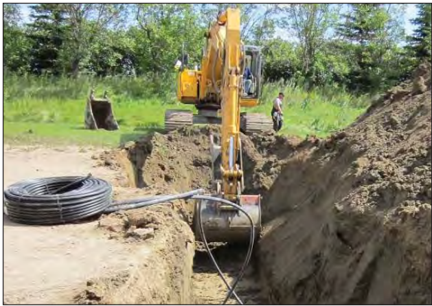
Figure 2. Installation of pipes for the ground source heating system installed in a grow-finish room.
