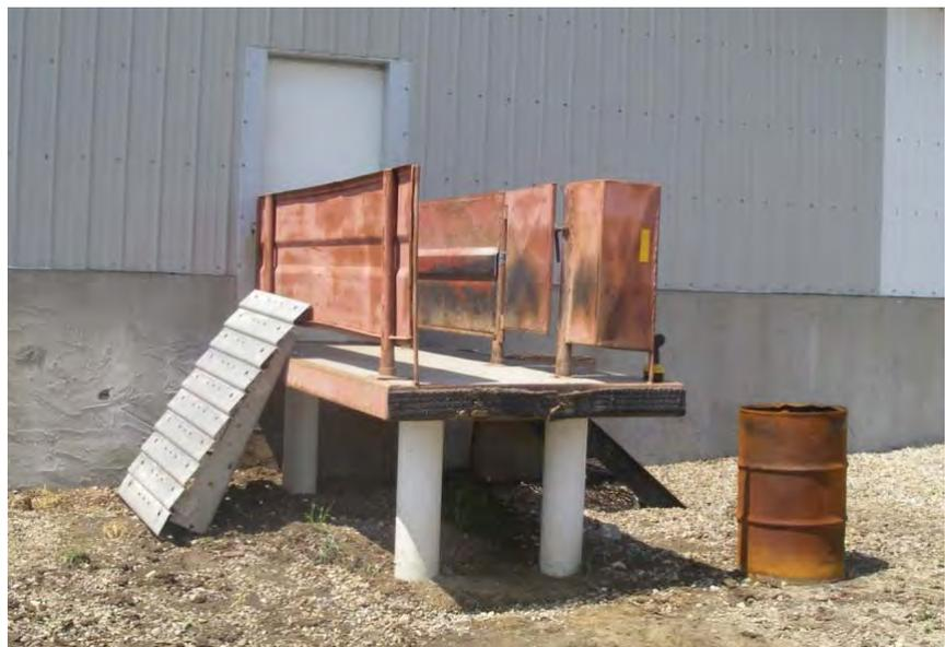
**Figure 3.** External loading ramp allows trucker to assist without entering barn. Note also the ramp extension (on the left) used to reduce the angle of internal truck ramp to the top deck
