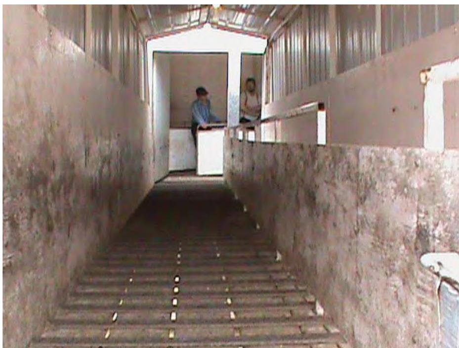
Figure 1. Covered hydraulic loading ramp with manway (looking down ramp from truck entry)
