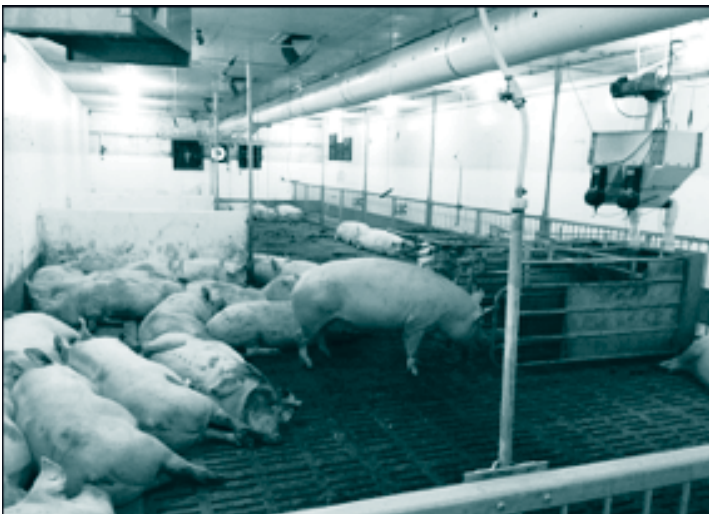
Figure 1. Photos of the control room with the existing (unmodified) ventilation system (A) and the treatment room with the air inlets on the opposite side (B) following the principle of a horizontal flow ventilation system. B – inset: wall air inlets installed in the treatment room.
