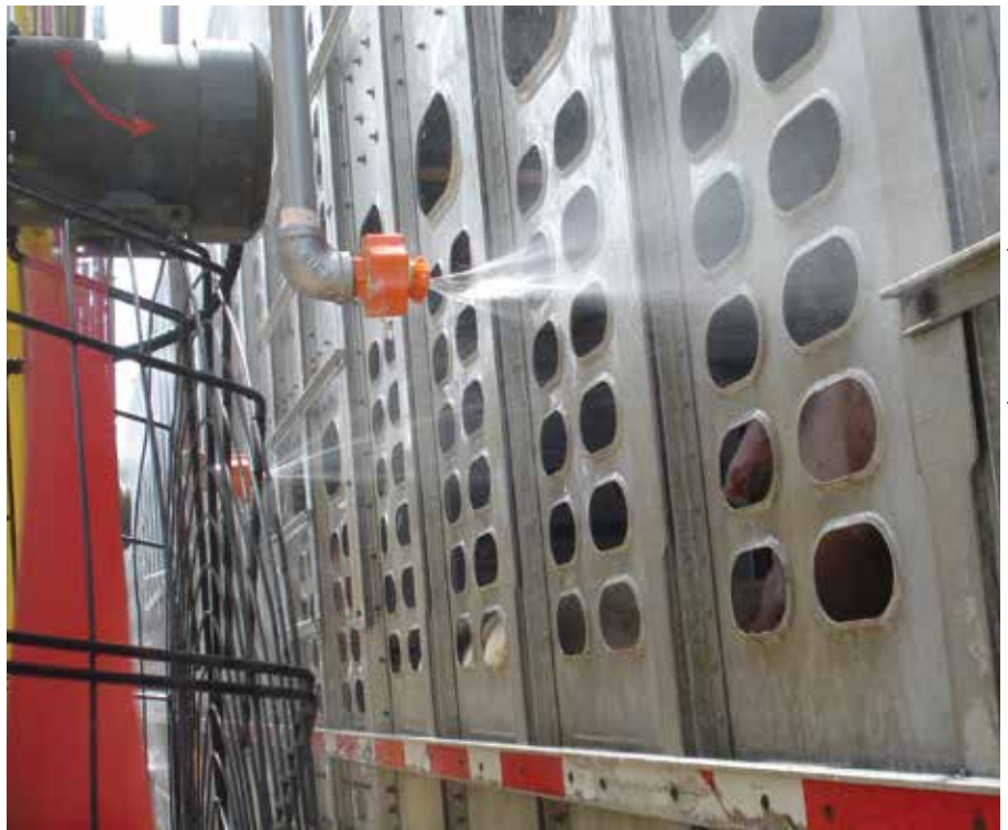
Researchers evaluated the impact of ventilation in warm conditions on the behaviour, physiology, and carcass and meat quality of pigs waiting to be unloaded at the slaughterhouse. Pictured here is a combined water sprinkling and ventilation system.
