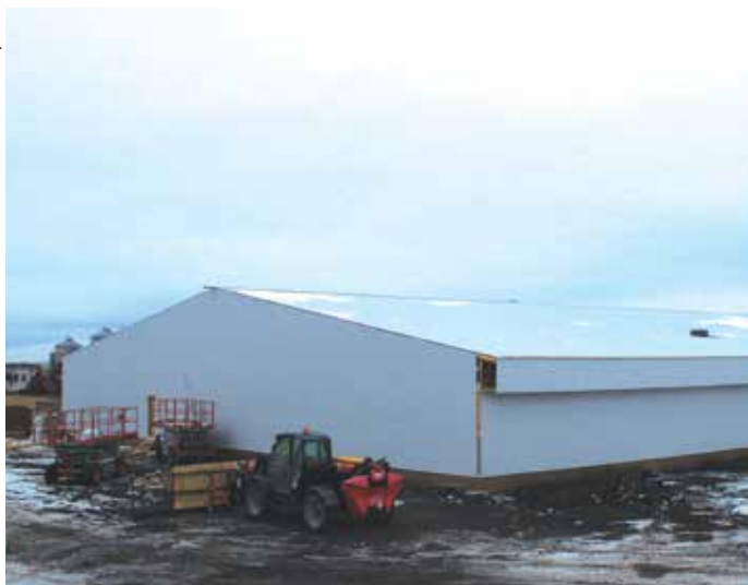
Jeroen Van Boekel is building a new sow barn in Rhineland, Man. to expand his operation's capacity to 5,000 pigs.
