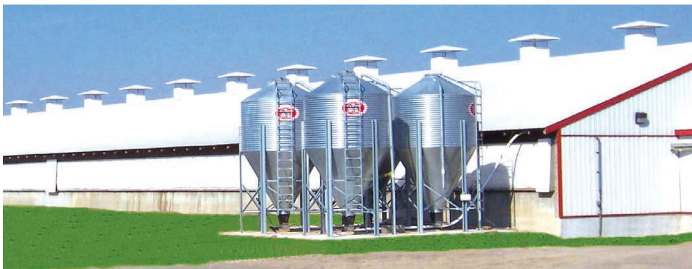
This barn has natural ventilation with an insulated curtain system.
