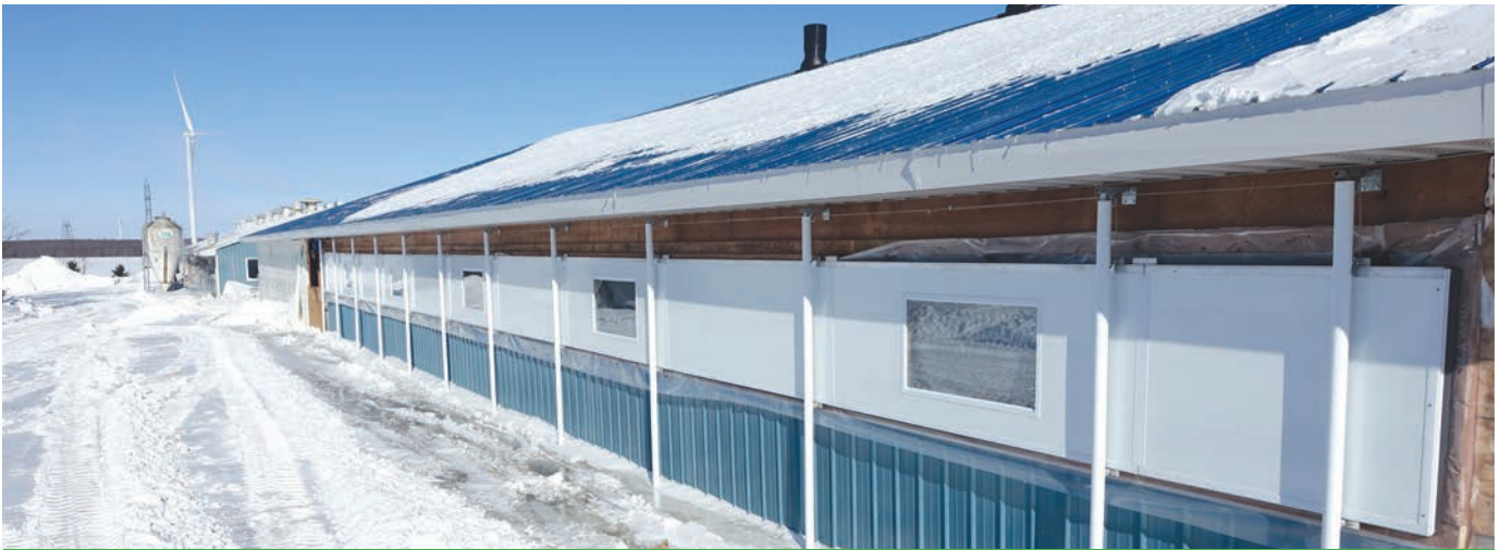
This barn has dual ventilation with a solid insulated panel system.
