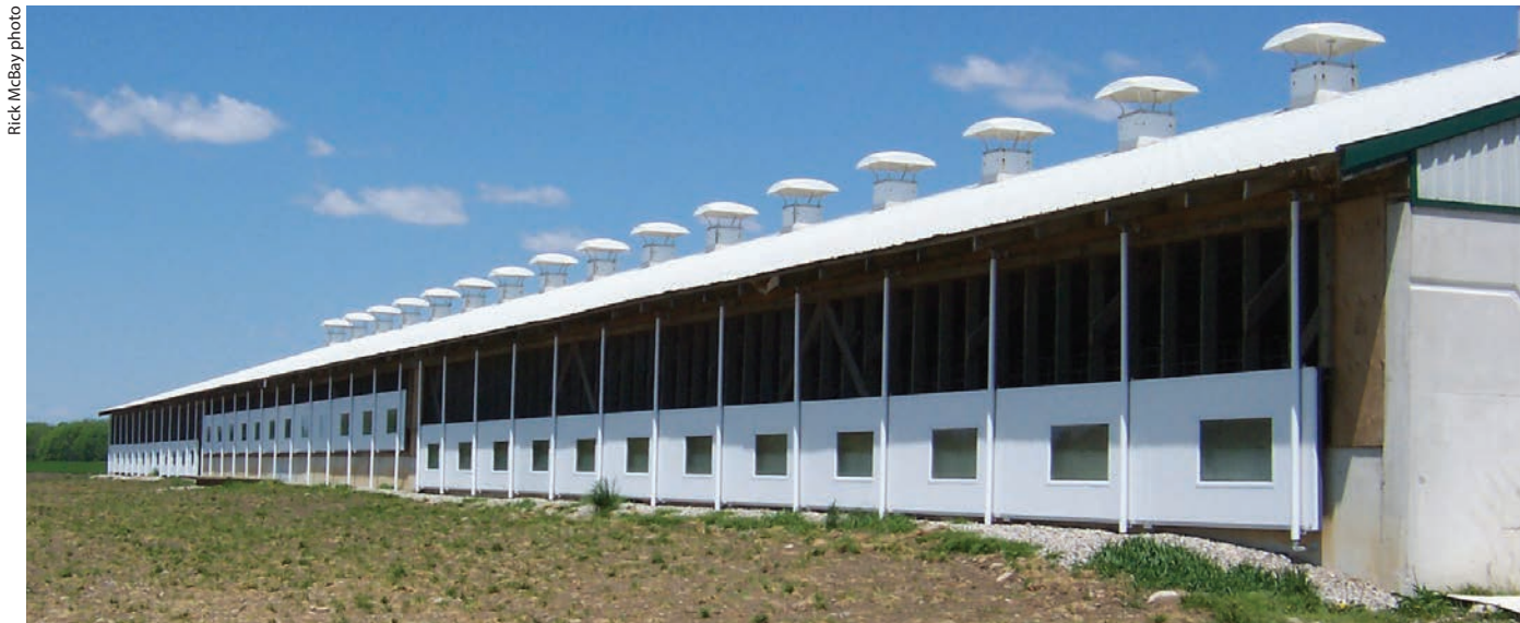
This barn has natural ventilation with a solid insulated panel system.
