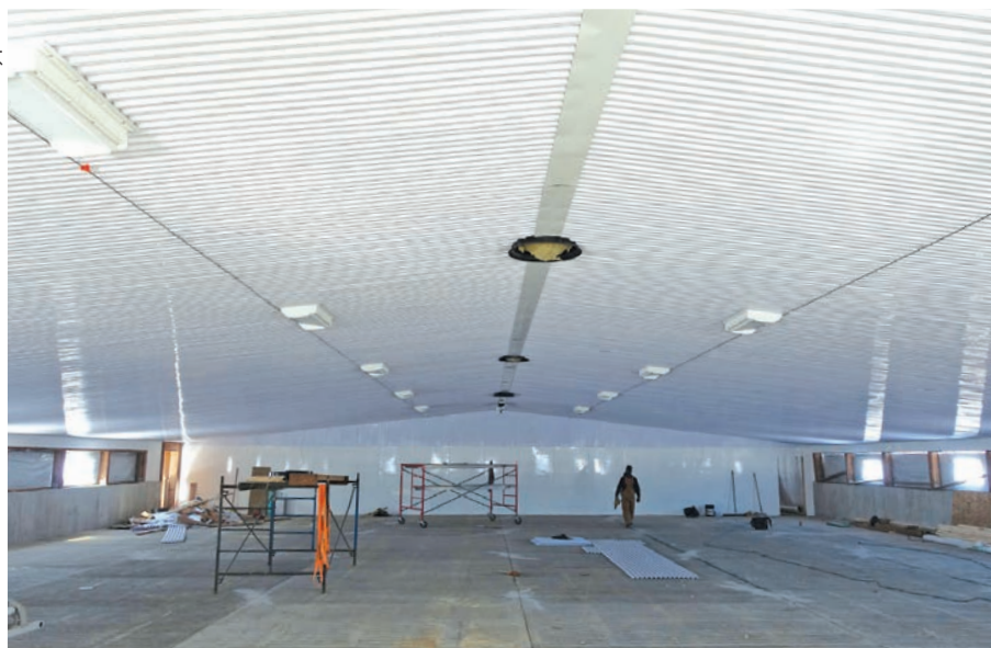
This barn has a dual ventilation system.
