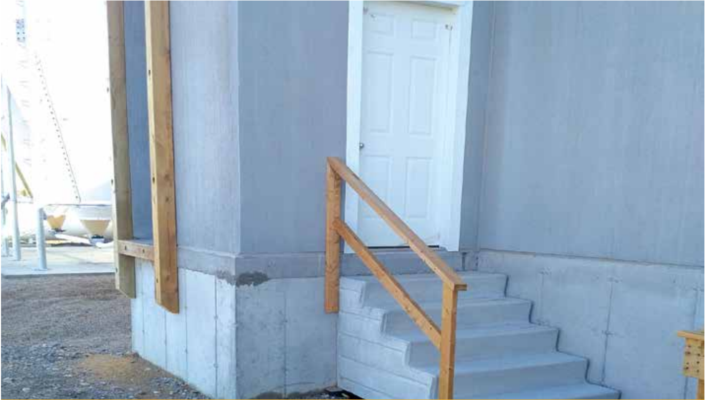
Stairs, rather than a ladder, make it easier for personnel to enter driver platforms.
