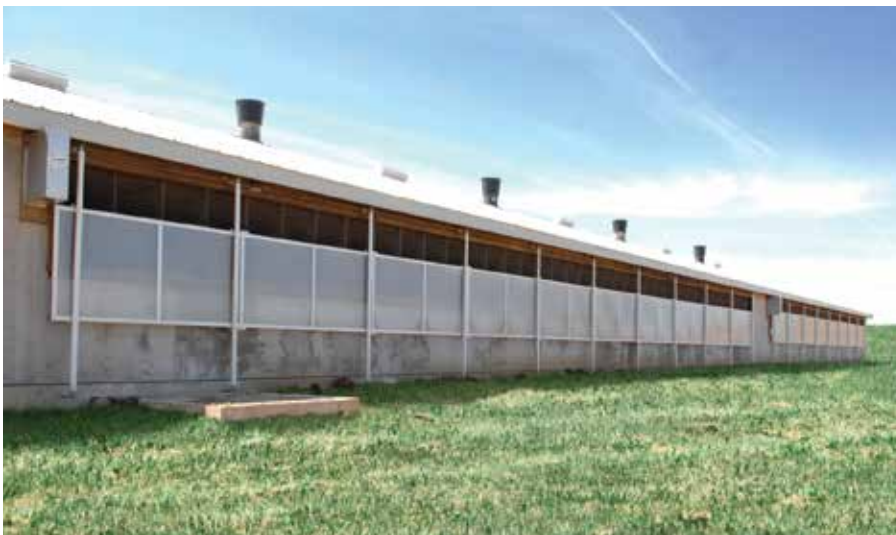
If natural light is important to you, then natural or dual ventilation systems that use translucent or clear panels are your best choice. The swine facility in this photo is dual ventilated.
