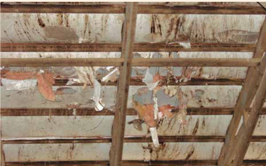
Birds and rodents will damage unprotected insulation.
