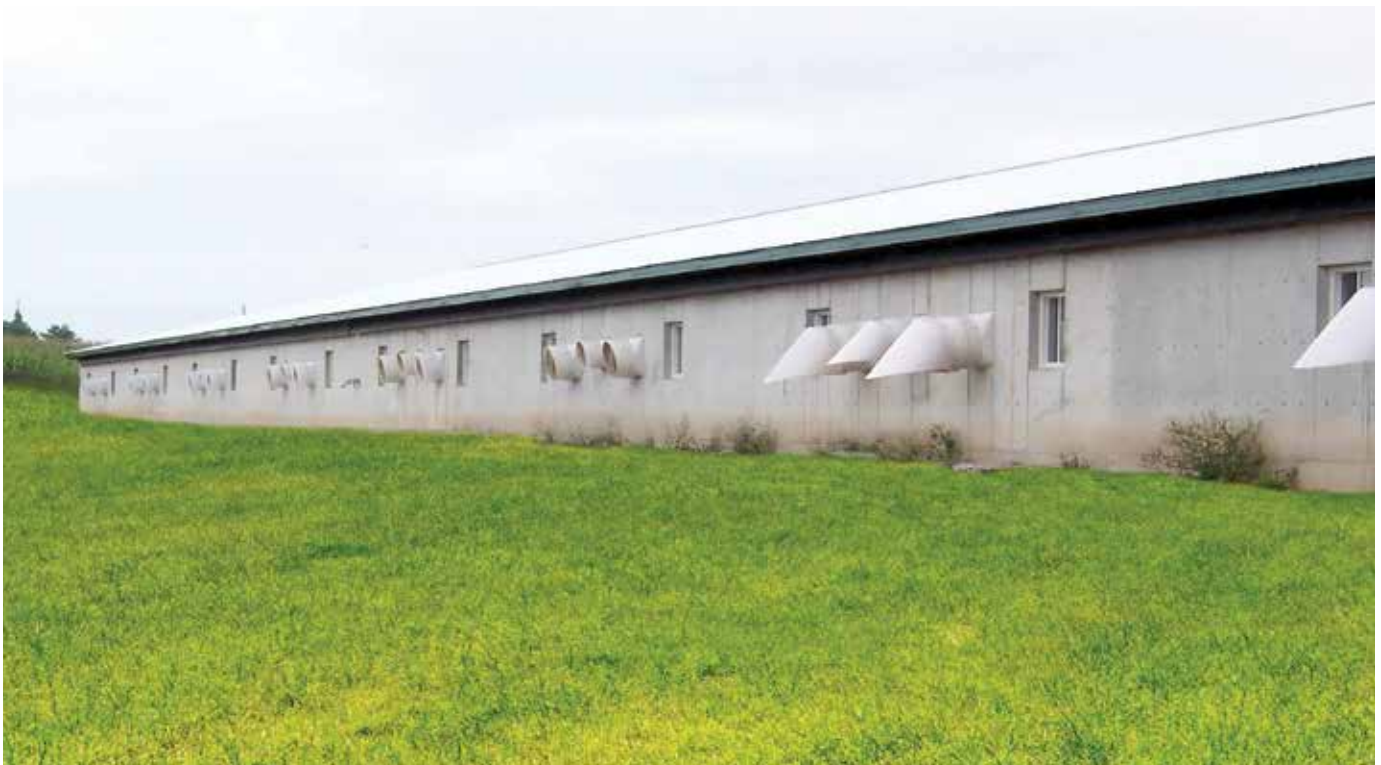
The tighter temperature control provided by power ventilation may ensure more comfort for animals with restricted movement in a stall design.
