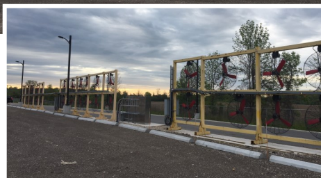
Fan banks installed at Conestoga Meats in Breslau, Ontario. Photos courtesy of Conestoga Meats
