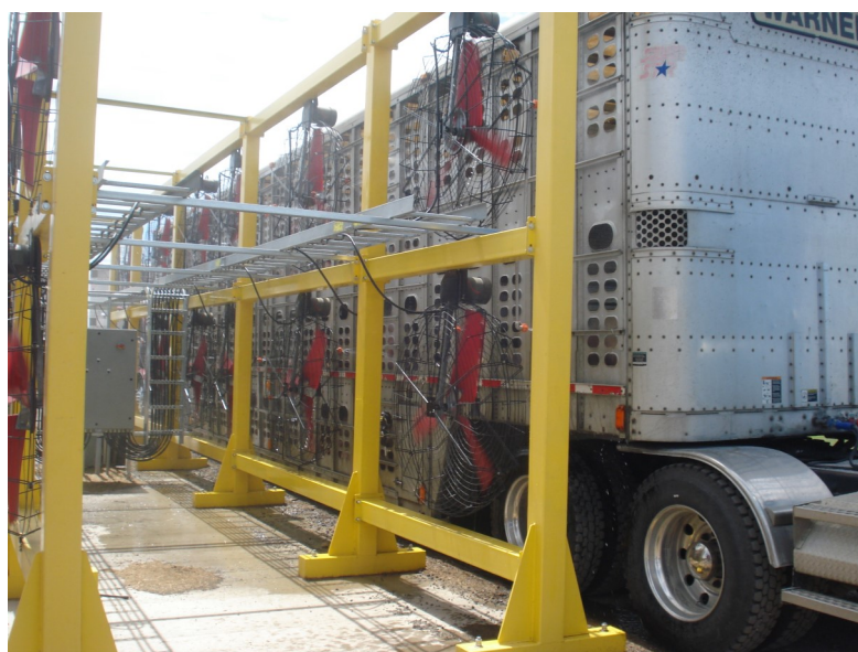
Ventilation system. Source: Sherbrooke Research and Development Centre, AAFC
