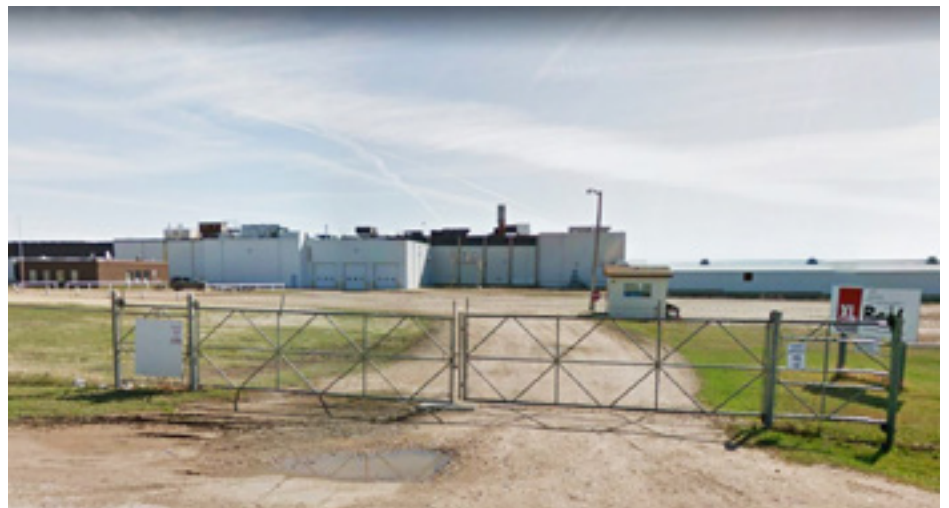
Donald’s Fine Foods will convert this former beef plant to a sow processing facility, opening next year.
