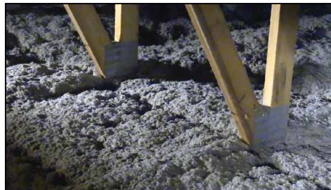
Insulation in the attic
