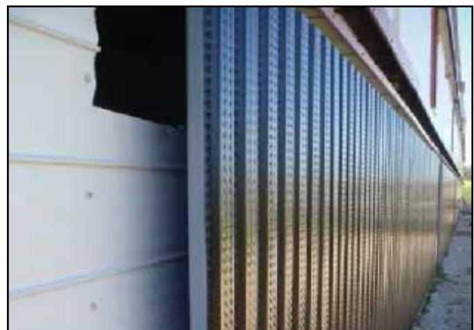
Close-up of a solar wall
