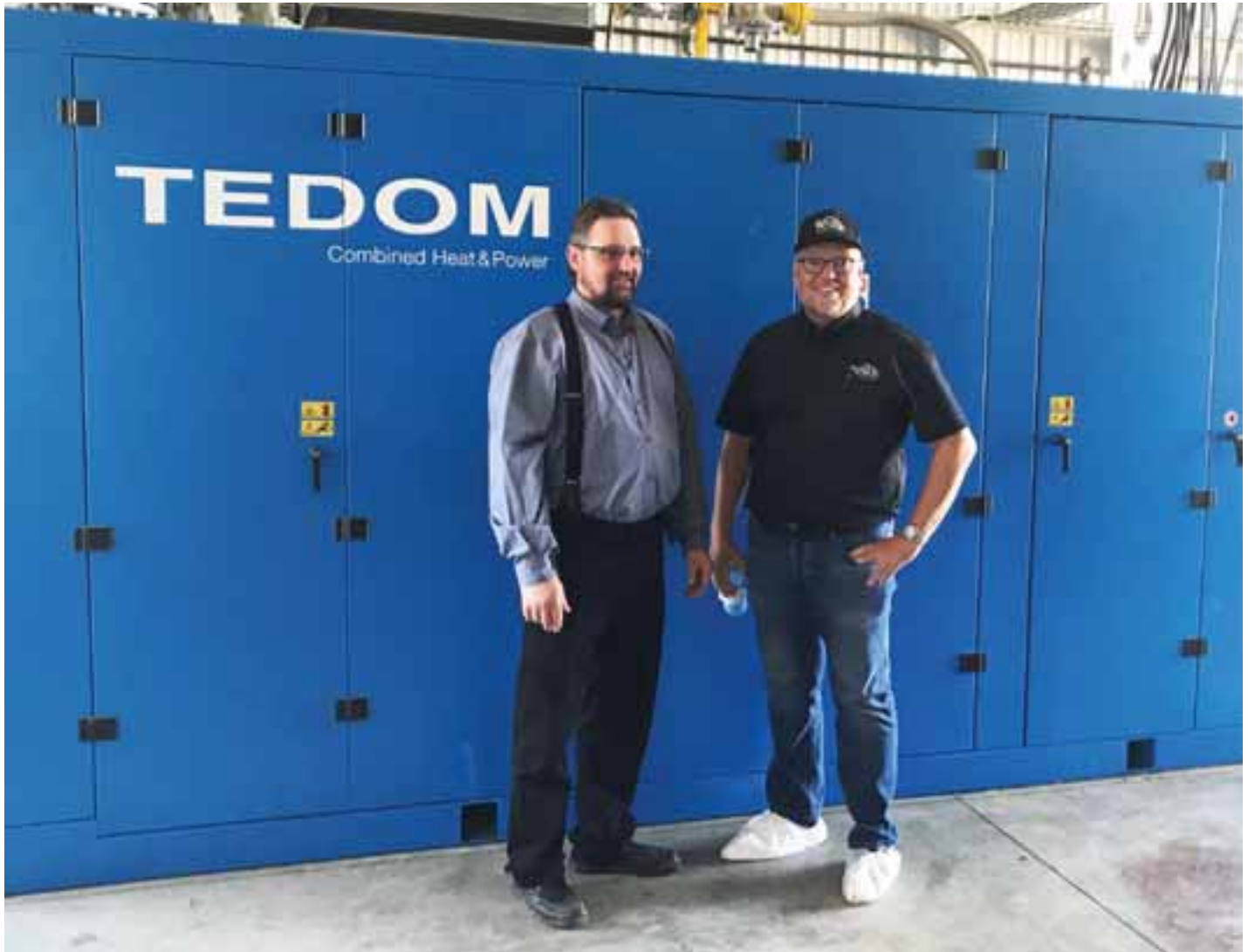
In August 2019, Hartland Colony installed a combined heat and power (CHP) unit in its hog barn. Since then, energy savings have allowed the unit to pay for itself, with many years of useful life still ahead. The technology was so successful that a second unit has since been purchased.
