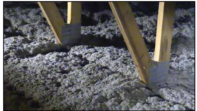
Insulation in the attic
