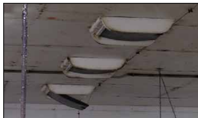
These air inlets should be adjusted and calibrated to introduce air uniformly
