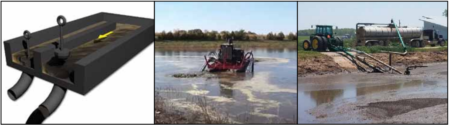
Energy is used when slurry is pumped from the barn to the outdoor storage facility (left), when slurry is agitated in the storage facility (middle), and when slurry is loaded and transported for field application (right).
